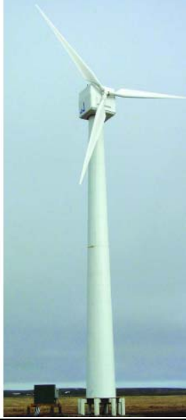
Vestas V27: 225 kW output, 27 meter rotor, pitch-controlled (power curve provided by Alaska Energy Authority).
