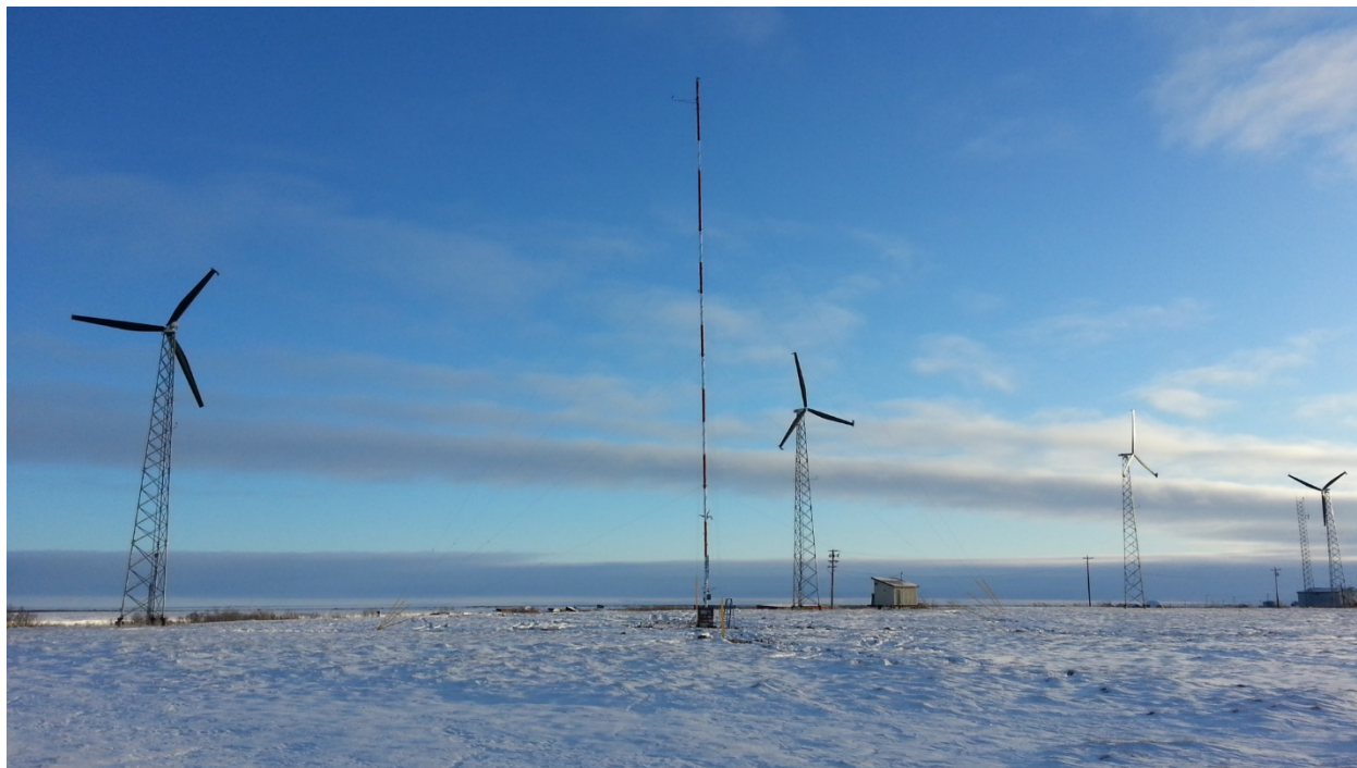
Selawik met tower and AOC15/50 wind turbines, photo by Douglas Vaught
