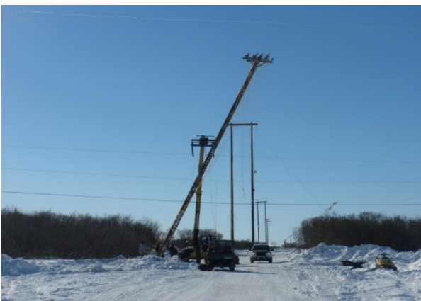
Installation of pole, attached to an H-pile.
