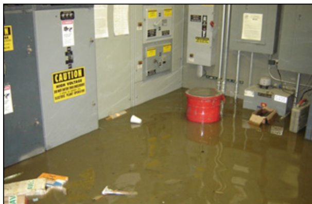
Water in the switchgear room, Emmonak.
