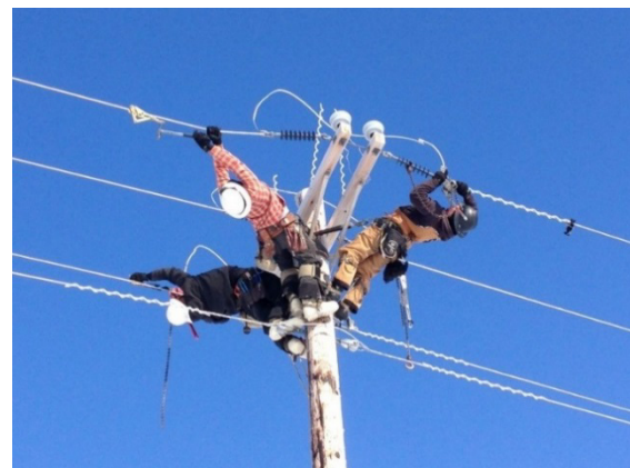
With most interties, manual labor can be used to tension the lines.
