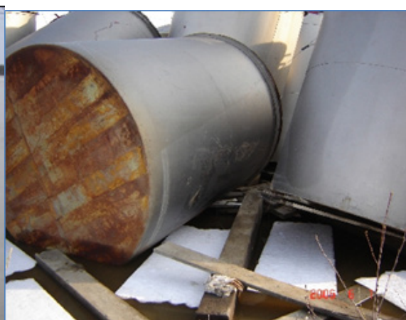
Fuel tanks floated off their foundations and toppled, Alakanuk.
