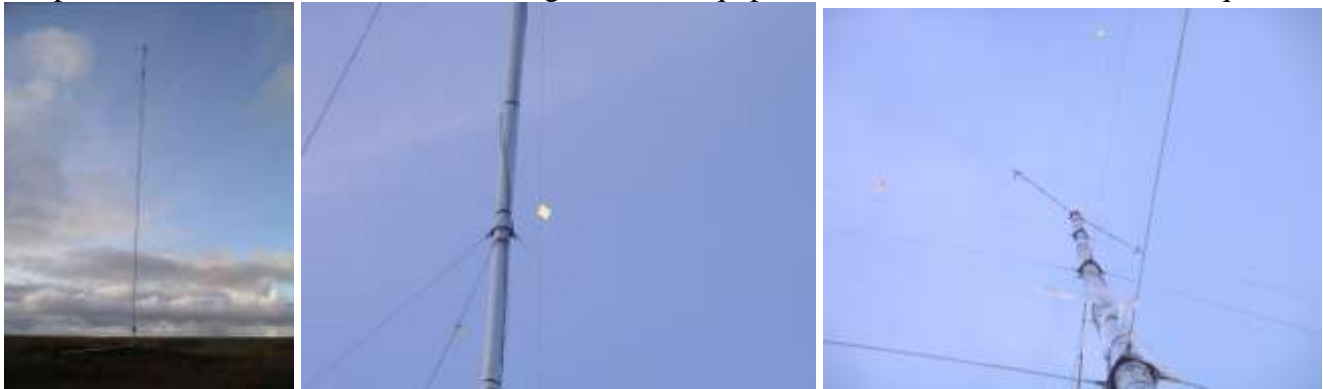
Figure 2. Photos of the Met Tower Installation in Nunam Iqua, AK
